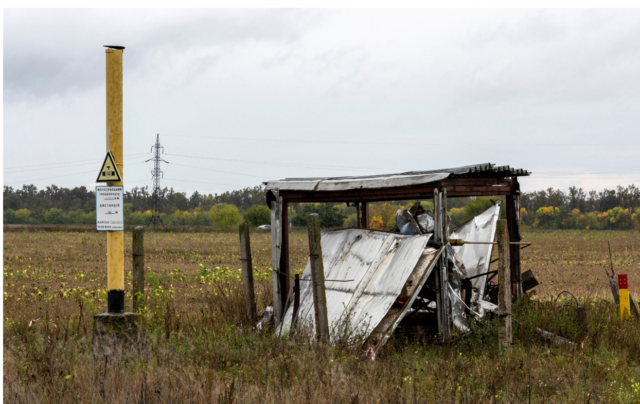
A gas pipeline valve station damaged by a shelling is seen near Balakliia, in Kharkiv region, Ukraine September 23, 2022. REUTERS/Umit Bektas
